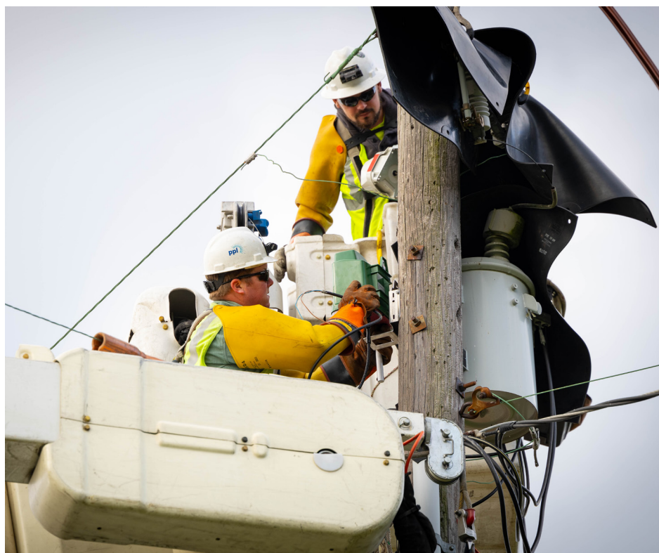
A team of lineworkers in Perry County installs a sensor on a line to optimize the ability to remotely and automatically reroute power, decreasing the number of customers affected by an outage and the length of time.
